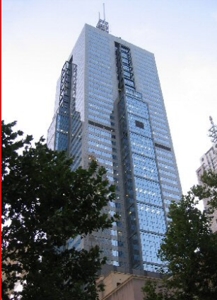
In building / PBX Integration
