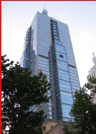
In building Emergency
